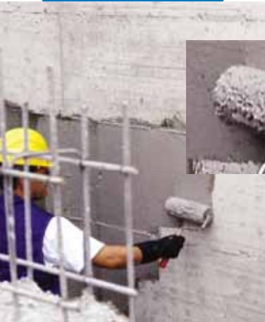
Waterproofing treatment applied by roller on a foundation wall
