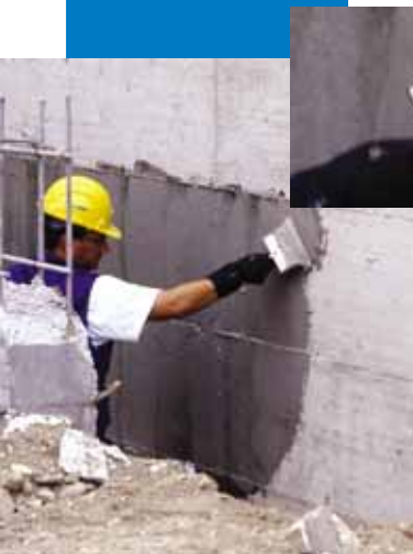
Waterproofing treatment applied by brush on a foundation wall
