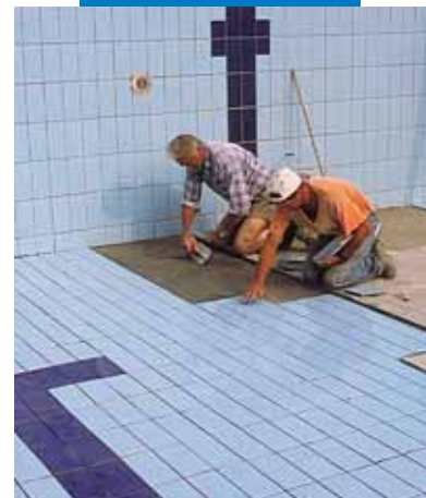
Laying of ceramic tiles on Mapelastic in a swimming pool
