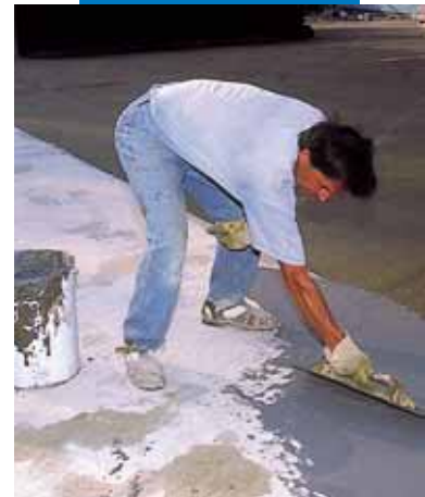
Waterproofing of a swimming pool with Mapelastic
