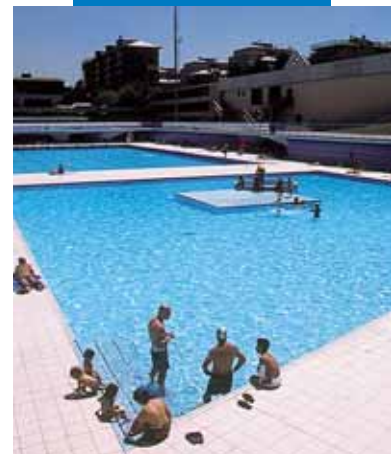
Swimming pool waterproofed with Mapelastic: Scarioni Leisure Centre - Milan - Italy
