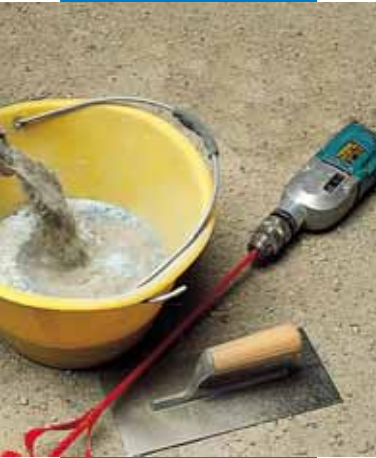
Mixing of Mapelastic with a mechanical mixer
